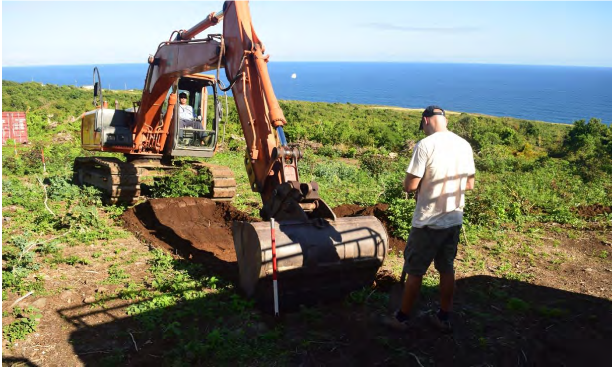
Figure 14: The tracked excavator excavating a trench (Photo: SECAR Staff).
