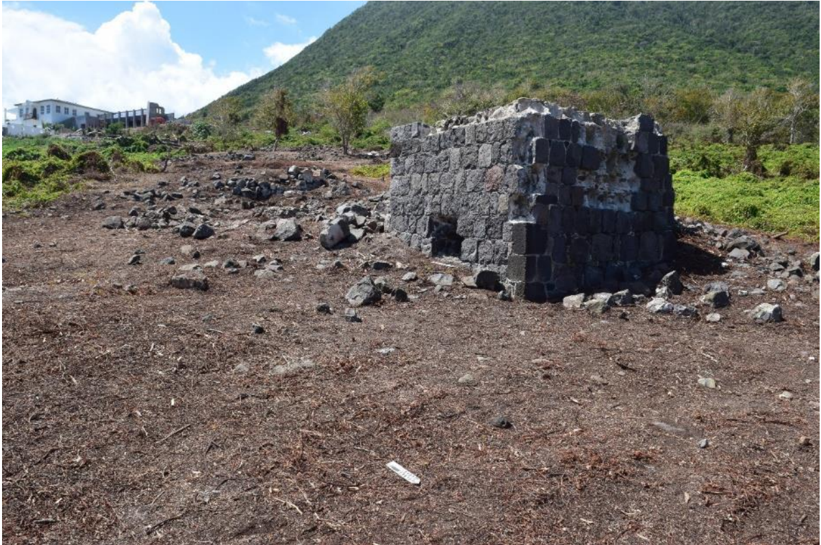
Figure 8: Overview of the industrial complex (Photo: SECAR Staff).
