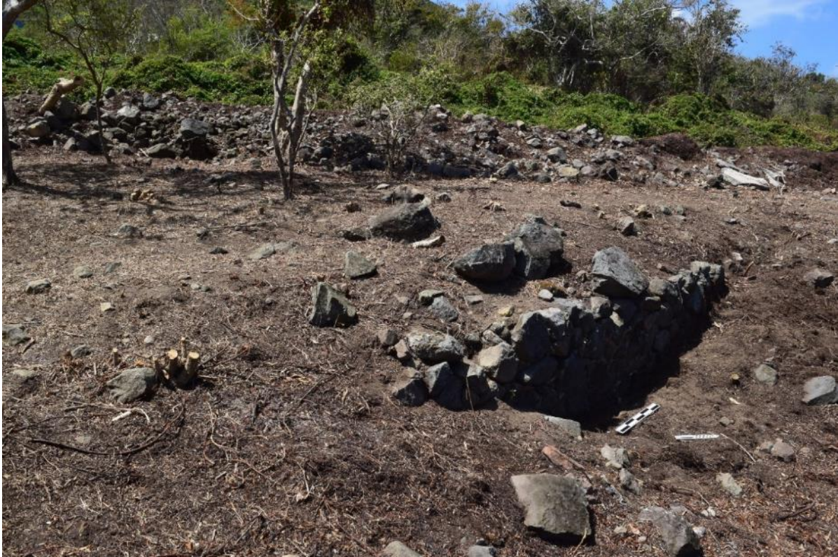
Figure 24: Retaining wall and plateau near the road (Photo: SECAR Staff).
